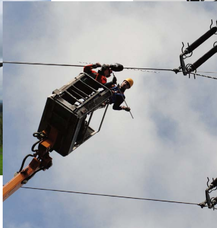
Mounting of sensor nodes at power line
