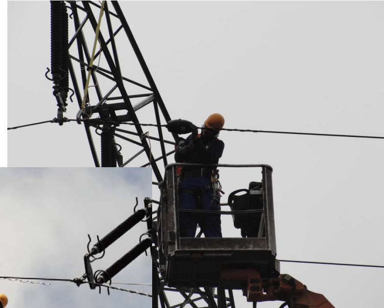
Mounting of sensor nodes at power line
