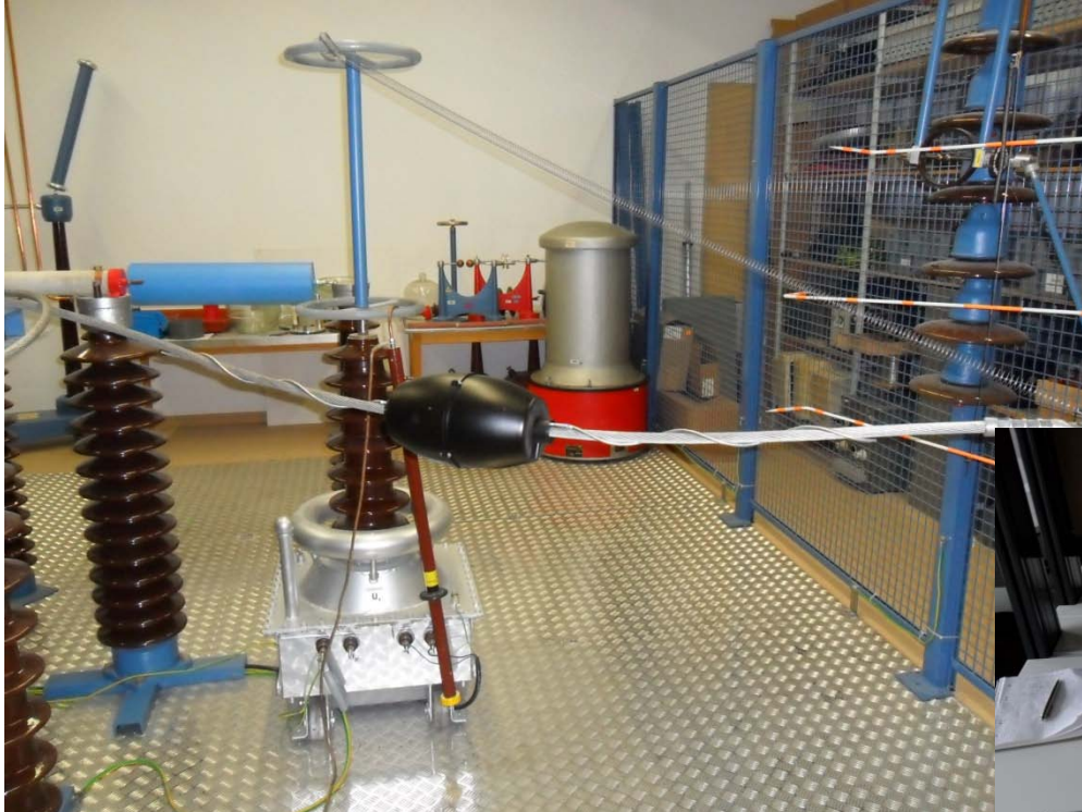
Function tests in high voltage laboratory (up to 110kV)
